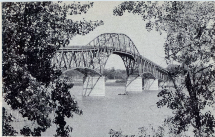
Highway Bridge at Port Henry
